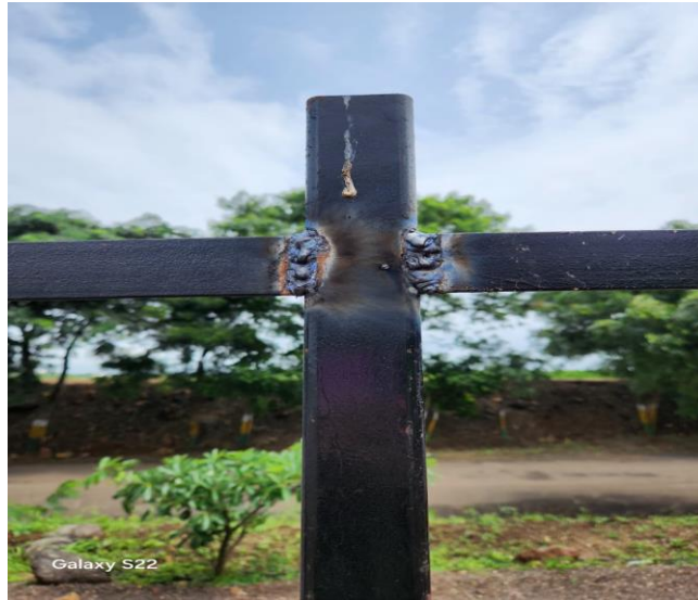
Photo6: Butt weld
