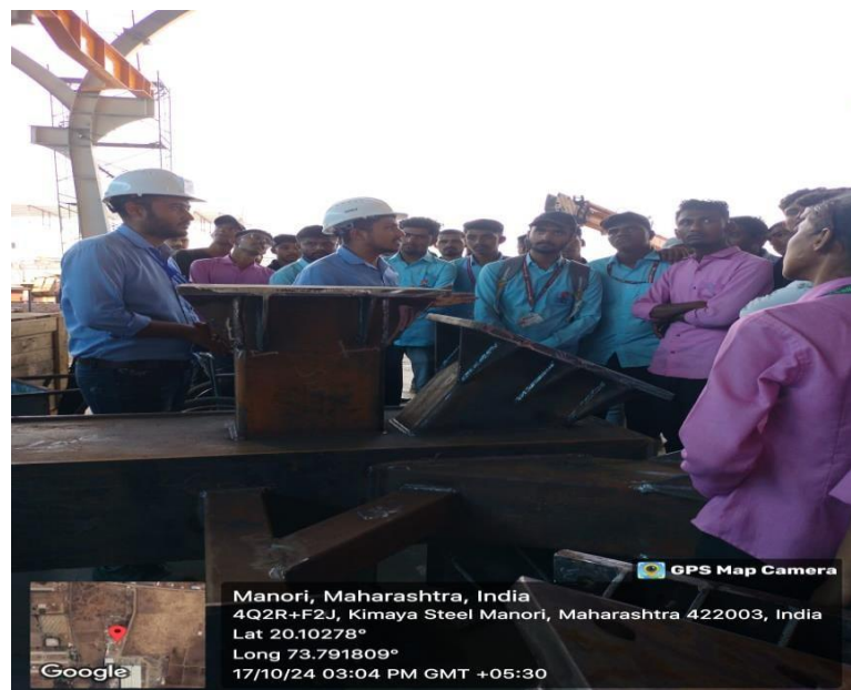
Photo 3: Students are learning the basics of Steel Structures
