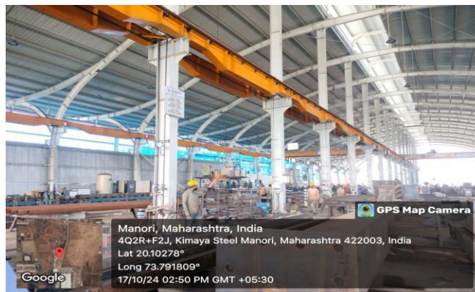
Photo: Gantry girder
