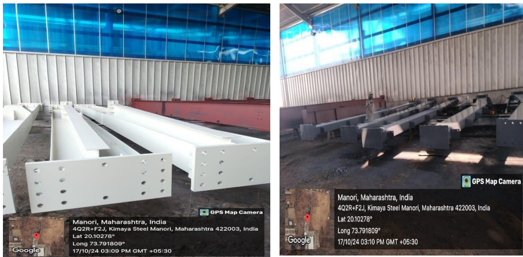
Photo 9: Student are learning the final coat of painting
