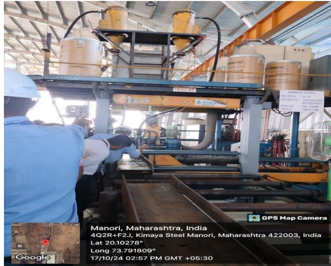
Photo 7: Students Learned welding on H Beam Welding Machine
