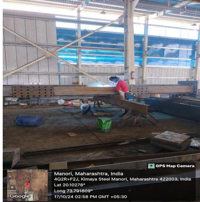
Photo 6: Process of Submerged-arc welding (SAW)
