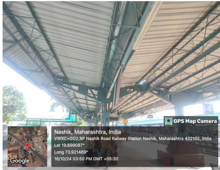
Photo 5: Components of Roof Truss
